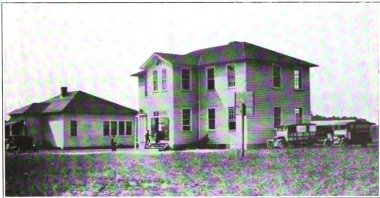
THE FIRST TWO BUILDINGS OF THE COUNTY TRAINING SCHOOL
